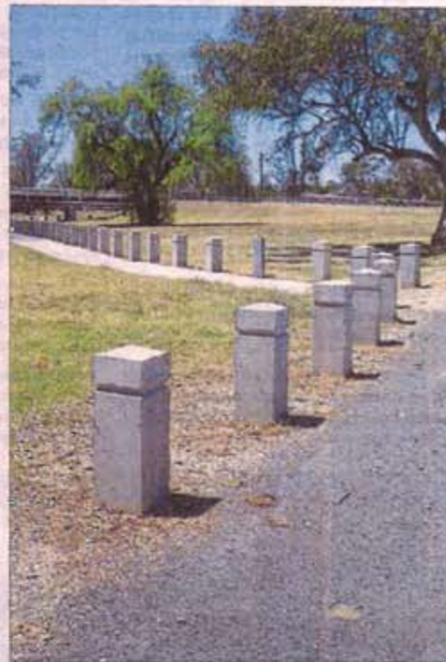
CEMENT bollards installed to protect the river banks.
