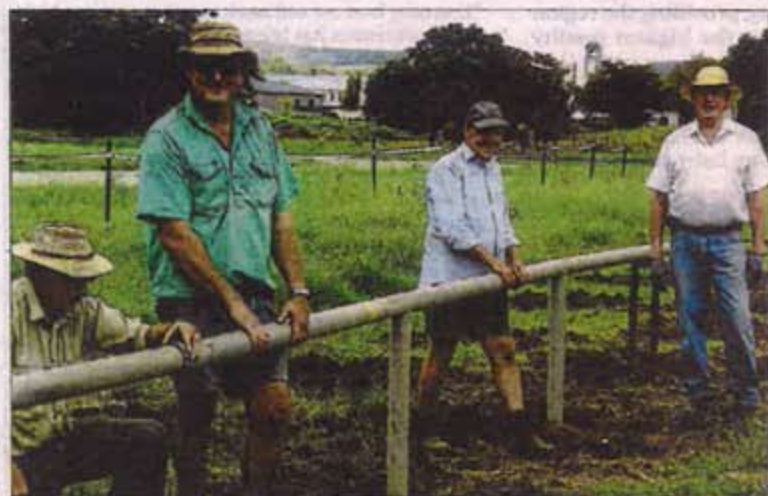
ROTARIANS working on the initial relocation of the fence around the playing fields early in the project. From left, Roger Corbett, Jamie Corbett, Rod Browne and Bob Laister.
